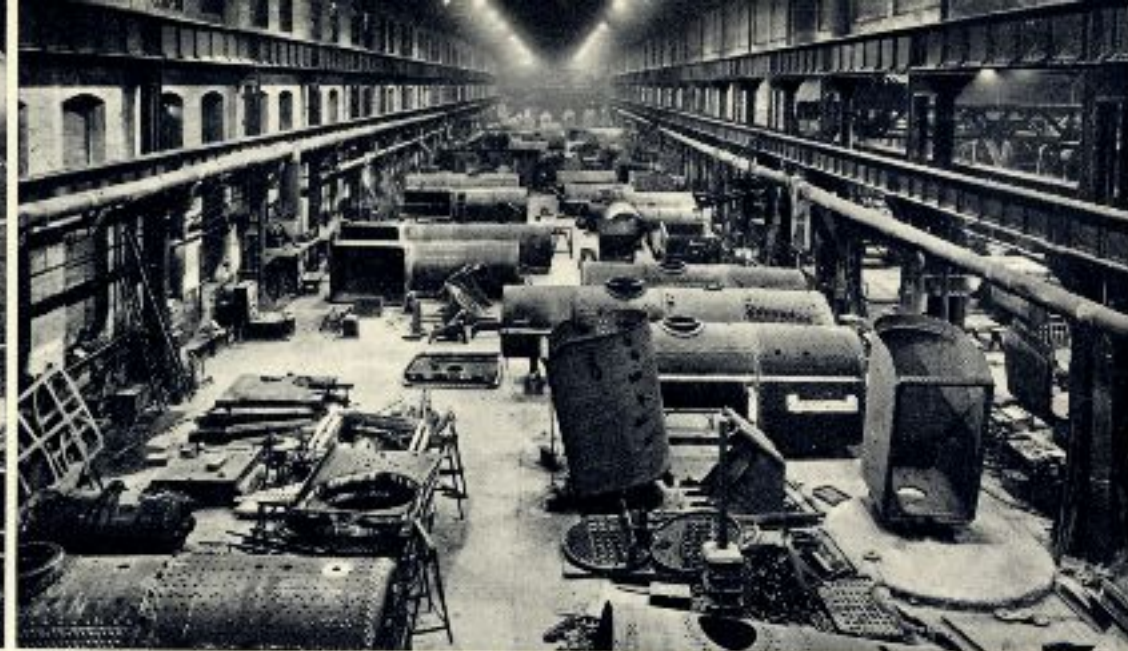
BOILER MAKING
